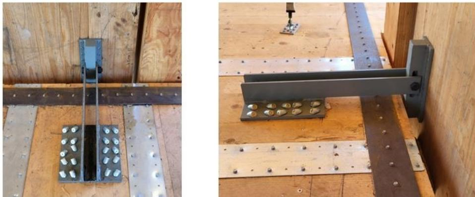
Left: Out-of-plane brace for the wall; Right: Complete wall-to-floor connection with shear key in the middle and braces on either side.
