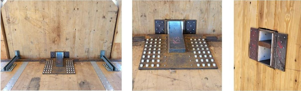
Left: Slotted shear key connection overview; Middle: Closeup view of fasteners; Right: Back side of shear key
