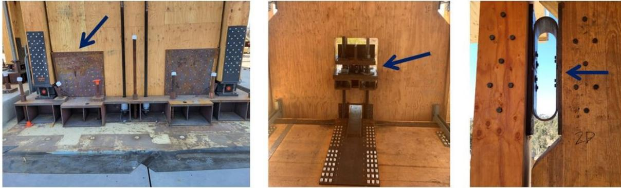
Left: Rocking wall with base shoes; Middle: Temporary post-tensioning for construction bracing; Right: UFP between wall panel and bounding column
