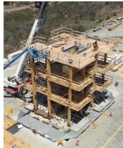
Left: Placing the south rocking wall; Middle: Site staff installing temporary post-tensioning; Right: First three stories complete
